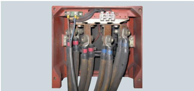
The power section voltage sensing inside the unit is floating with respect to the electronics (electrically isolated).
